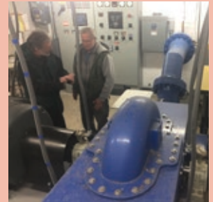
Mike Holecsek of Aeon Renewable Energy and City electrician Mark Heider discuss the workings of the City's rebuilt hydro plant.
