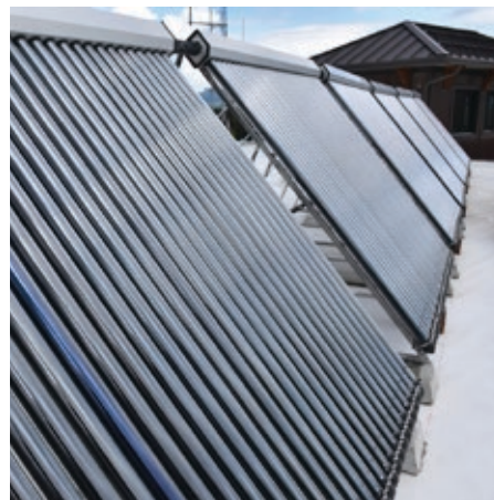
The Emergency Services Building uses solar thermal collectors to heat some of its hot water.
