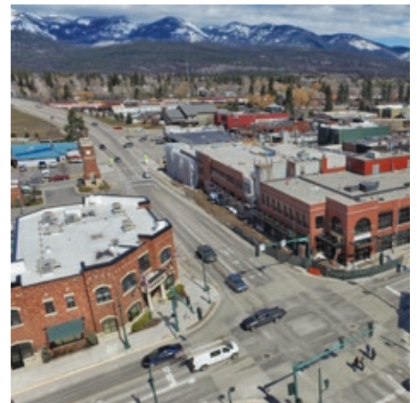
Intersections along US 93 and Wisconsin Avenue are projected to have significant congestion by the year 2030.
