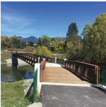
Three bike/pedestrian bridges have been built connecting trails along the Whitefish River.
